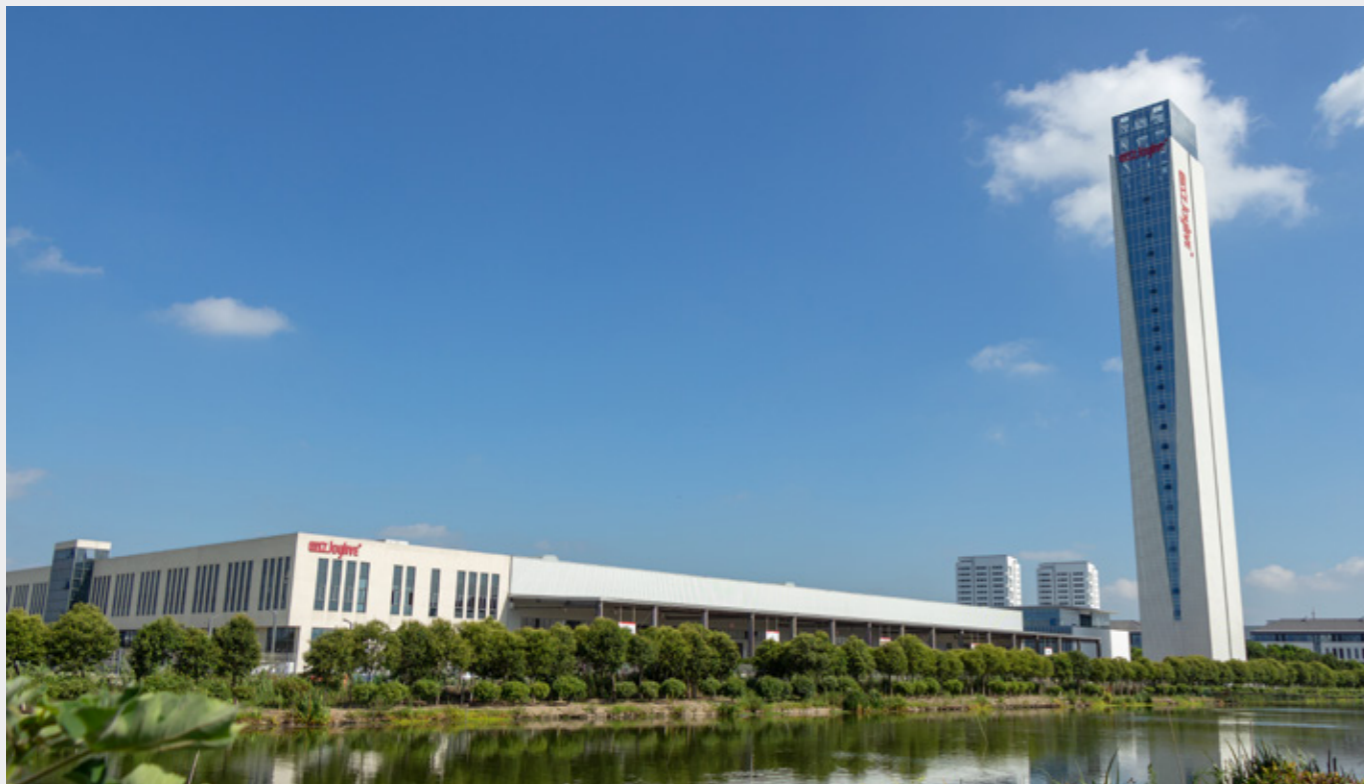
70, 000 m2 area manufacturing factory with 118 m height test tower
